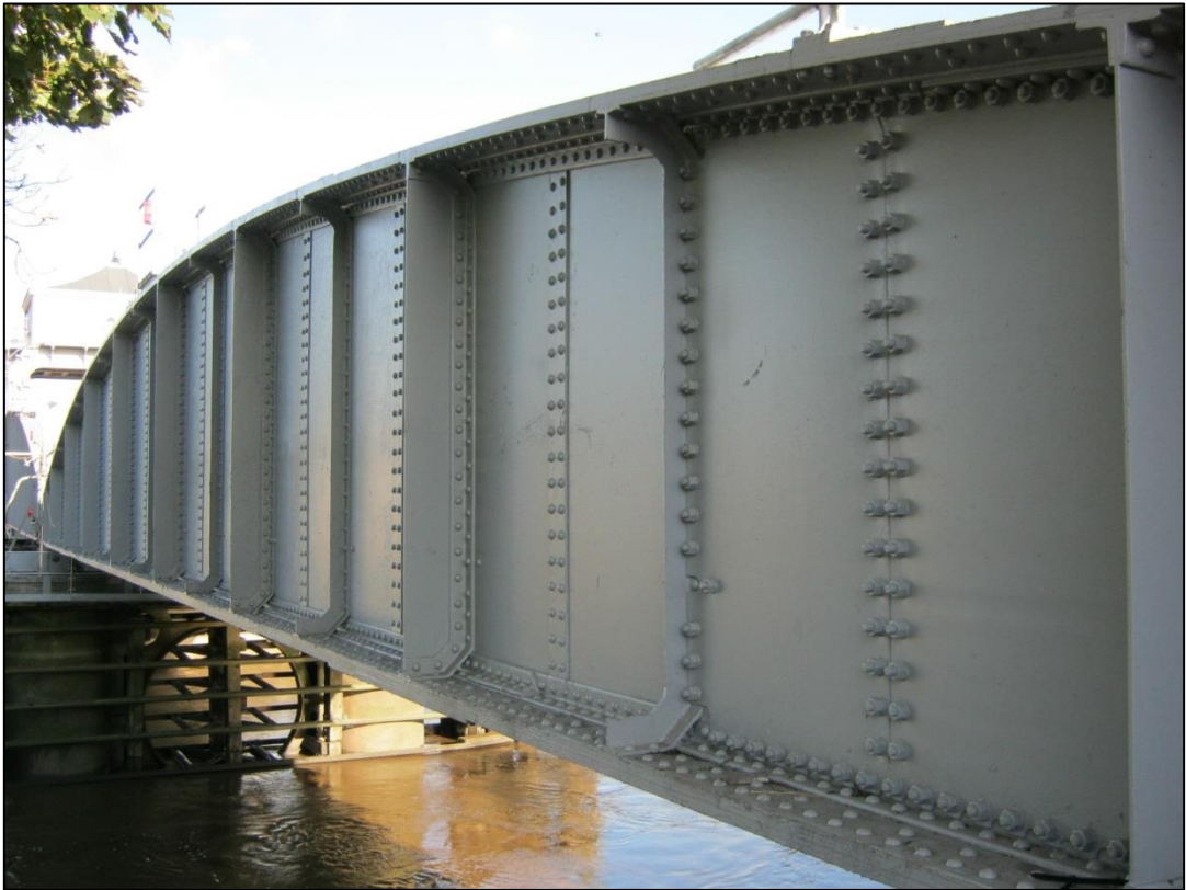
Photo 11 – After Application of Termarust
