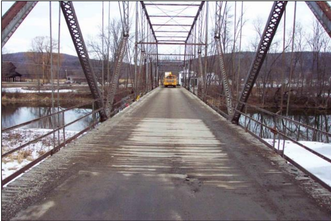
Photo 4 – Prior to Painting
