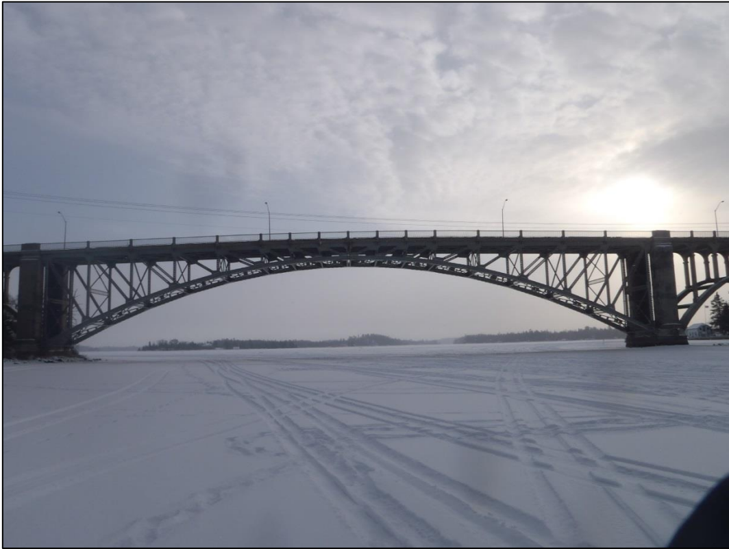
Photo 6 – Elevation on Bridge
